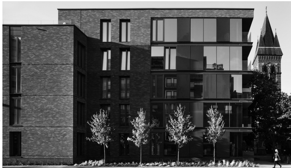
Cortesia Dolphin Living
